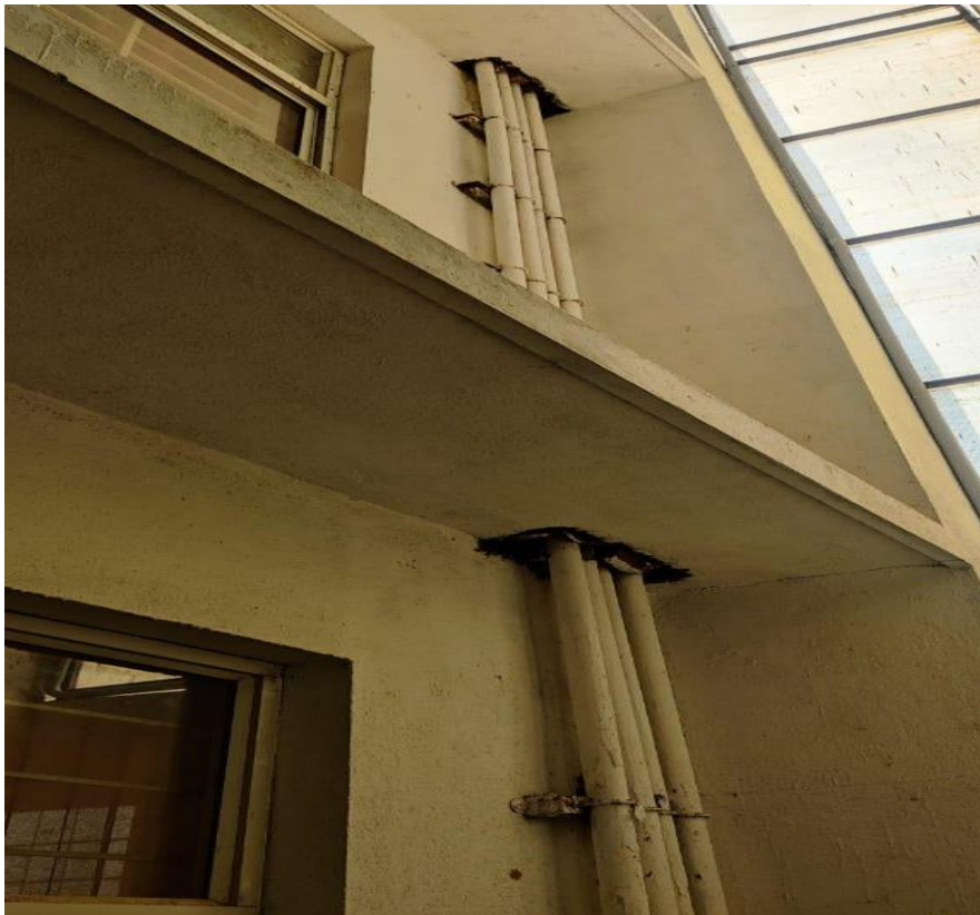
4. PHOTOGRAPHS SHOWING RAIN WATER TRANSFERRED TO MAIN DISTRIBUTION TANK THROUGH DISTRIBUTION PIPES
