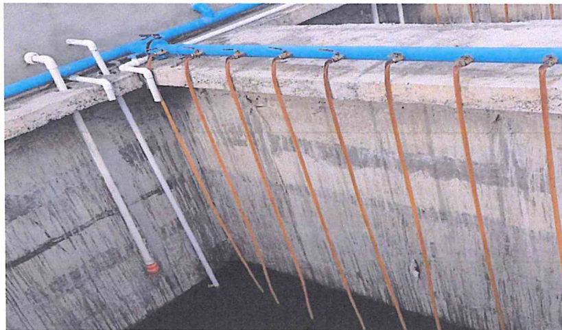
4. WATER COLLECTING TANKS
